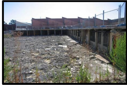
Warehouse Demolition – February 2006
