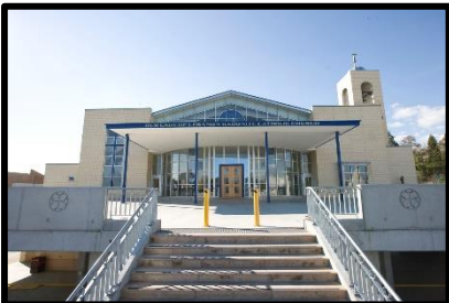
Church Completed – March 2008
