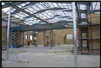
Church Brick Work – May 2007
