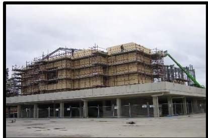
Church Brick Work – May 2007
