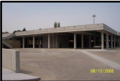
Level One Complete – December 2006
