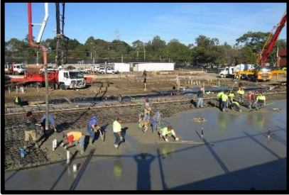
Concreting Begins – April 2006
